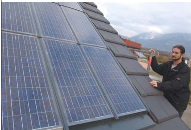
Roof-integrated photovoltaic panels (INES).
