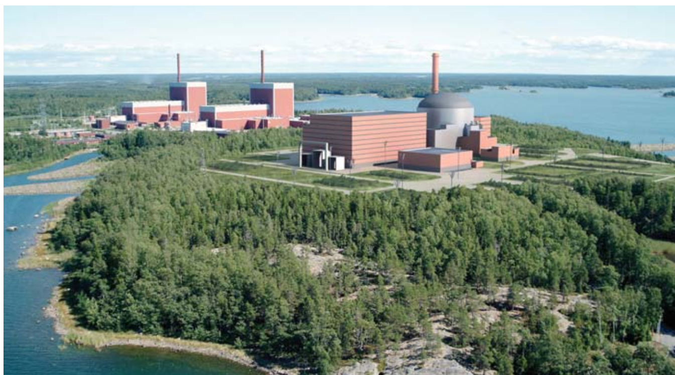
The Olkiluoto (Finland) site, showing, in the foreground (computer-generated imagery), the first European third-generation nuclear reactor (EPR), to be built by Framatome-ANP (Areva Group) and Siemens (for the conventional section), as forerunner to the initial series model, to be built by French electricity utility EDF at Flamanville (Manche département). In the background, the two second-generation reactors operated by TVO may be seen.
