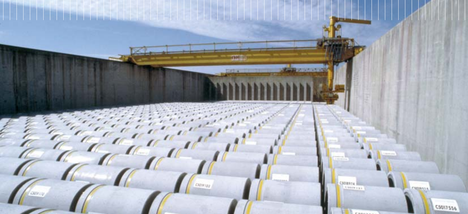
Cemented waste package in the solid waste storage workshop (EDS: Entreposage des déchets solides ) at the Areva NC (Cogema) plant, at La Hague (Manche département).
