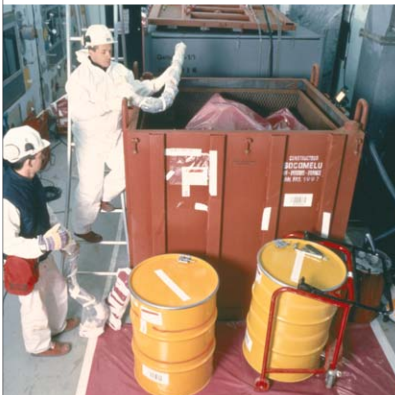
Containerization of products from the dismantling of Brennilis power station (Finistère département, Western France).
