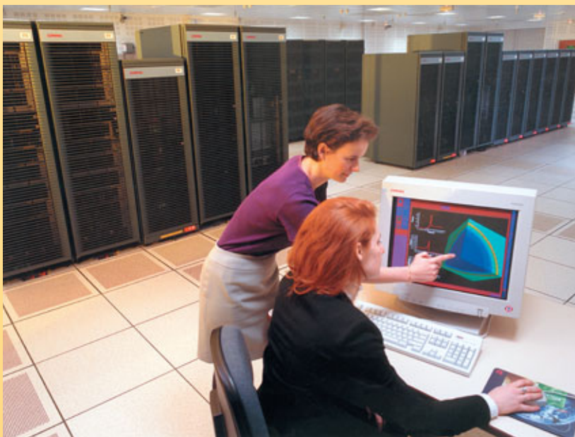
Installed at CEA (DAM-Ile de France Center) in December 2001, the TERA machine designed by Compaq (now HP) has for its basic element a mini-computer with 4 x 1-GHz processors sharing 4 GB of memory and giving a total performance of 8 Gflops. These basic elements are interconnected through a fast network designed by Quadrics Ltd. A synchronization operation across all 2,560 processors is completed in under 25 microseconds. The overall file system offers 50 terabytes of storage space for input/output with an aggregate bandwidth of 7.5 GB/s.
