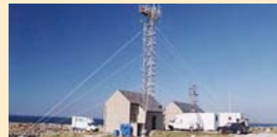
The Mace Head monitoring station, Ireland.
