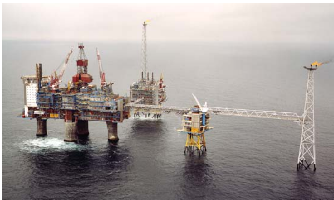
Sleipner Platform, in the North Sea, operated by Norwegian group Statoil. A CO 2 injection experiment was carried out beneath the seabed, in this oilfield.
