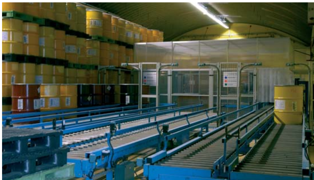
Storage hall for drums of waste at CEA Saclay, awaiting consignment to ANDRA (in yellow) or CentraCo (red-brown), after characterization on the automated CAMDICES line.
