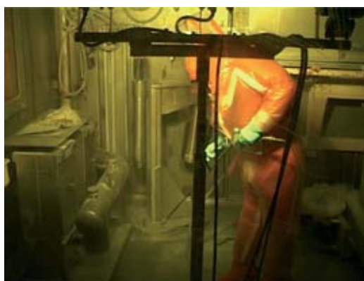
Decontamination by means of a vacuumable gel of a cell in the ISAI installation, at CEA's Marcoule Center.
