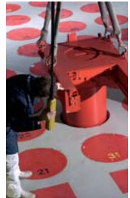
Waste storage hall at CEA/Saclay, comprising 100 wells, each with a 10-drum capacity.
