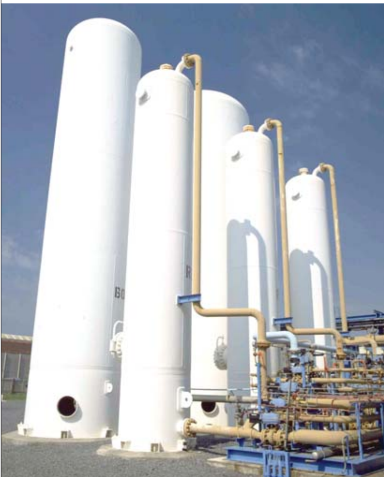
Hydrogen PSA production unit operated by Air liquide's Group, at Waziers (Nord département, northern France).
