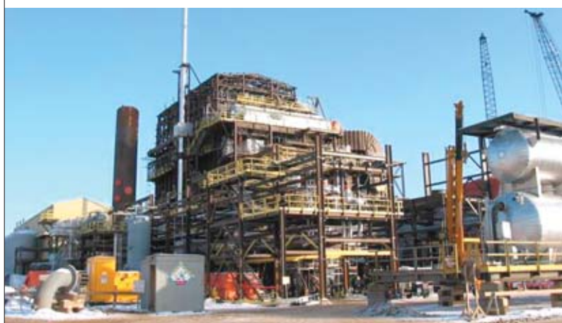
The steam reforming unit built by Technip for Syncrude Canada. Over a single line, this has an output of 223,000 Nm 3 /h hydrogen, and a further 75 MW electricity.
