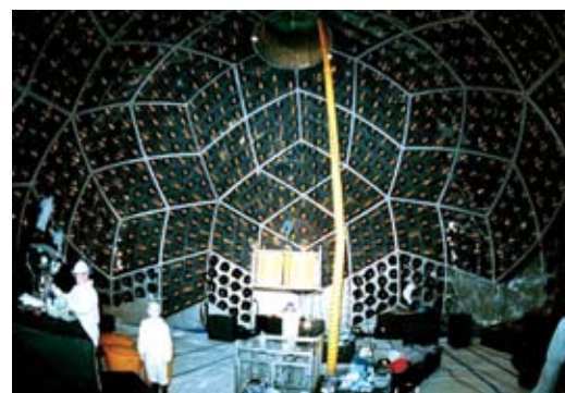
A model (top) of the entire detector complex for the KamLAND experiment. Bottom: a view inside the detector, as the photomultiplier tubes were being installed.
