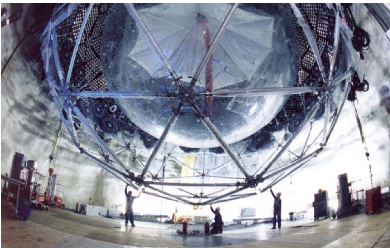
A view of the target of the Sudbury Neutrino Observatory (SNO), during construction, comprising 1,000 tonnes of heavy water, contained in an acrylic-plastic vessel. This volume is monitored by 9,600 detectors, borne on the metal structure.
