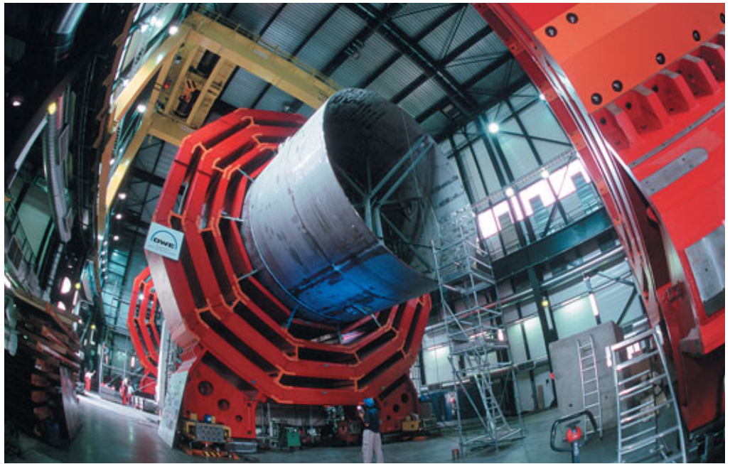
Installation of the CMS detector at the incipient LHC. The outer magnet ring has been inserted down the axis of the detector.
