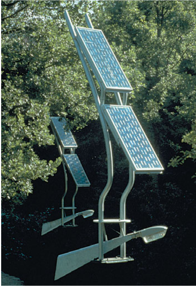
Lamp posts with individual photovoltaic cell power supply in Antibes (Alpes-Maritimes).
