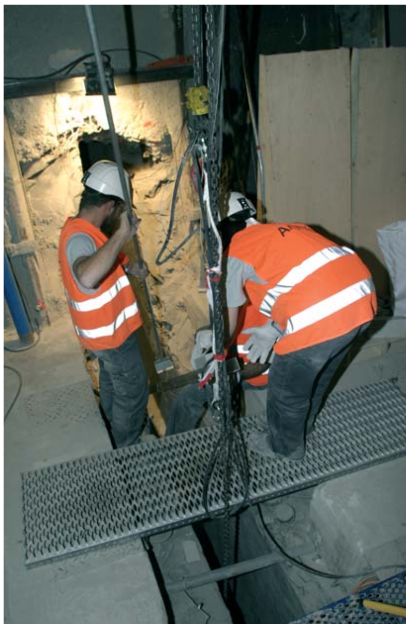
Constructed at a depth of 500 m, at the boundary of the Meuse and Haute-Marne départements (North-Eastern France), in an argillaceous layer with an age of 150 million years, ANDRA's Underground Research Laboratory is a multidisciplinary research instrument, for the investigation of disposal conditions in a deep geological environment for long-lived radioactive waste. Shown here, an experiment carried out at the bottom of the shaft.
