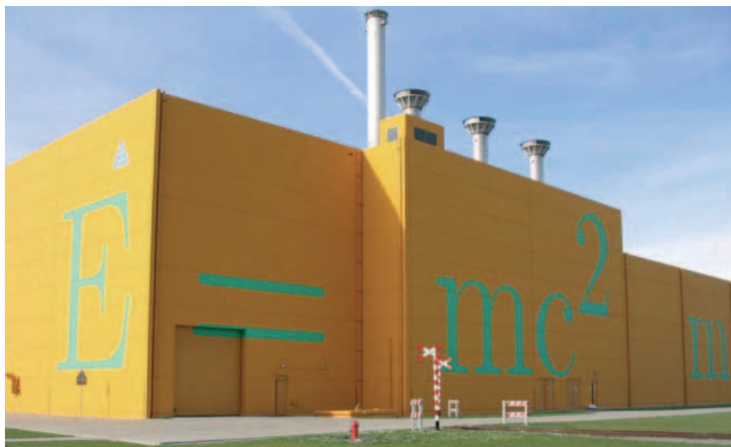
The HABOG high-level waste and spent fuel storage facility, opened in September 2003 at Borsele (Netherlands).
