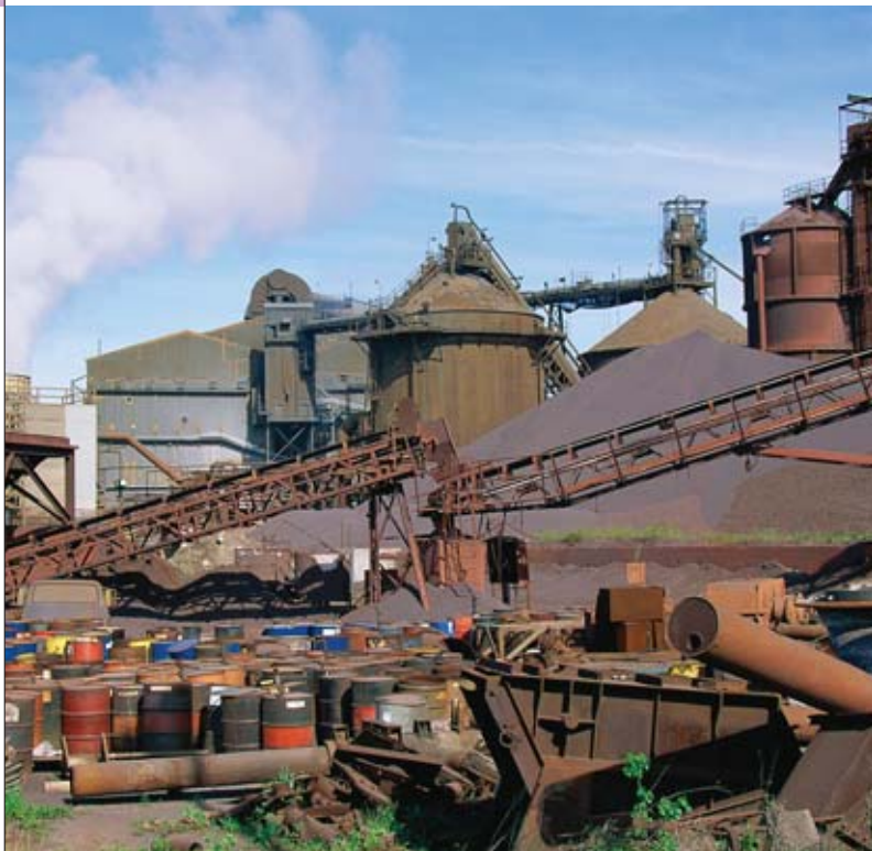
Storage of materials on an old industrial site. Practically all the metals recognised as carcinogenic in man were identified in heavily exposed workers in the past.
