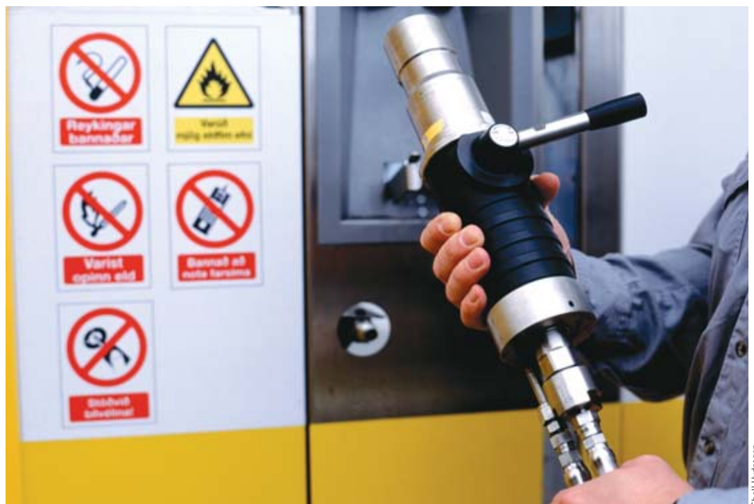
Hydrogen nozzle in a service-station run by Shell Hydrogen in Iceland, under the aegis of the ECTOS Program. Identification and control of the risks associated to this fuel must bring it to the same safety level as any other.
