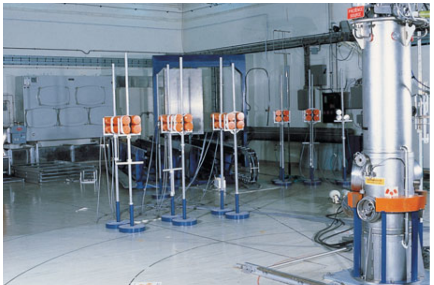
Testing Edac accident detection system sensors around the core of the Silène reactor.
