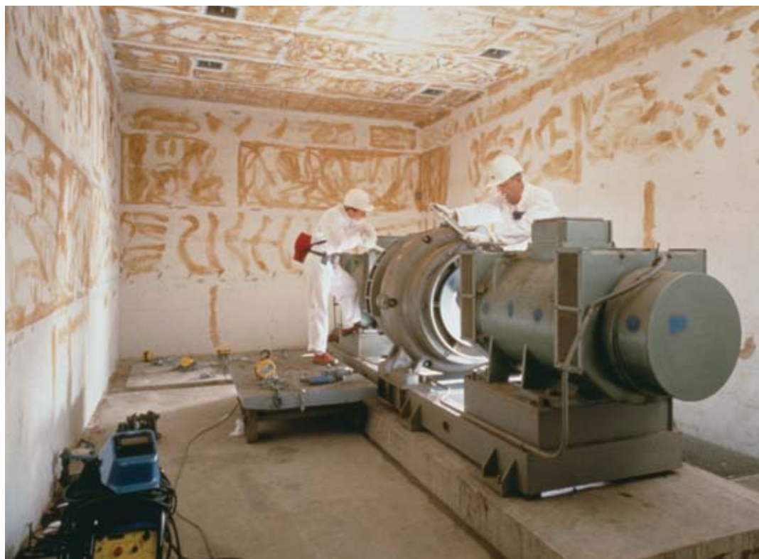
Dismantling the Brennilis power station (Finistère). The disassembly of old plant can expose workers to elements in unfamiliar physicochemical forms.
