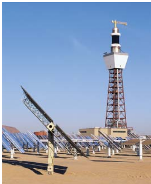
Tower power station built by Luz Solar International Corp., in California, one of the main commercial developments in the area of solar thermodynamic energy at the end of the 20th century.
