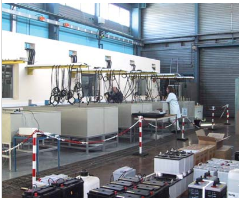
Testing hall at Cadarache, where CEA is investigating behavior and optimization of batteries coupled to photovoltaic modules.
