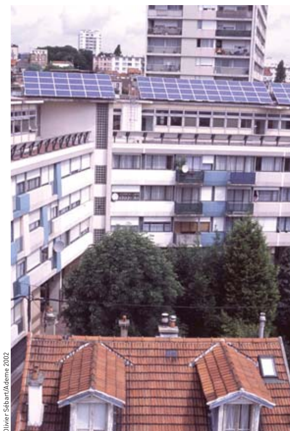
Added-value use of renewable energies favors improved building energy efficiency indicators in housing. Part of the domestic water for these apartments in a social housing block in Montreuil (Seine-Saint-Denis département , Paris Region) is heated by 220 m 2 of solar photovoltaic collector panels installed on the roof.
