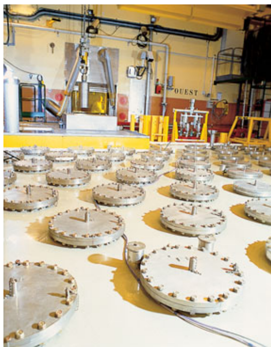
Shaft heads containing various types of fuel in the Cascad dry-storage bunker facility at CEA/Cadarache, the current reference design concept.
