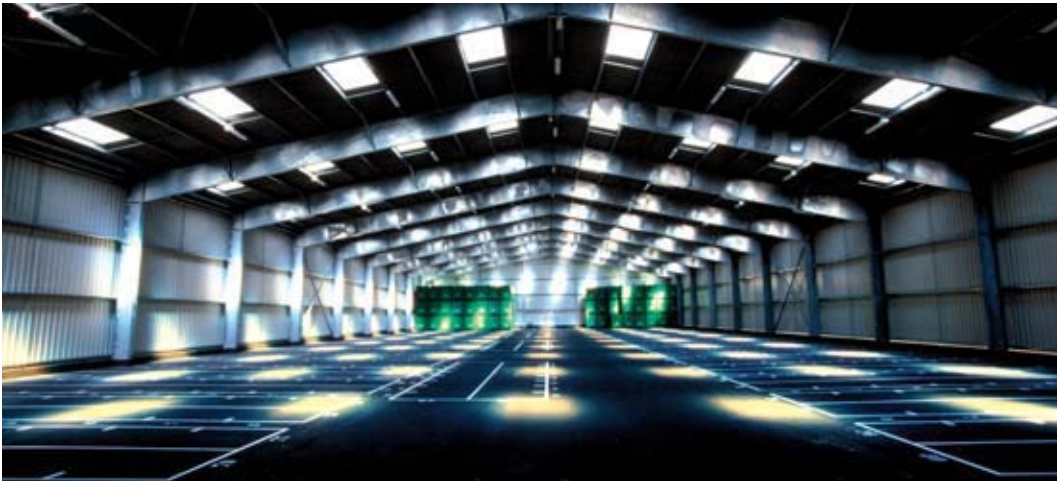
Depleted uranium (U 3 O 8 ) container storage hall at the Bessines (Haute-Vienne département , southwestern France) industrial site.
