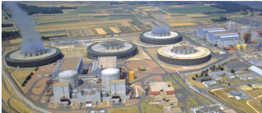
The four PWR units of EDF's Avoine power station, near Chinon (central France), belong to the second generation of nuclear reactors.
