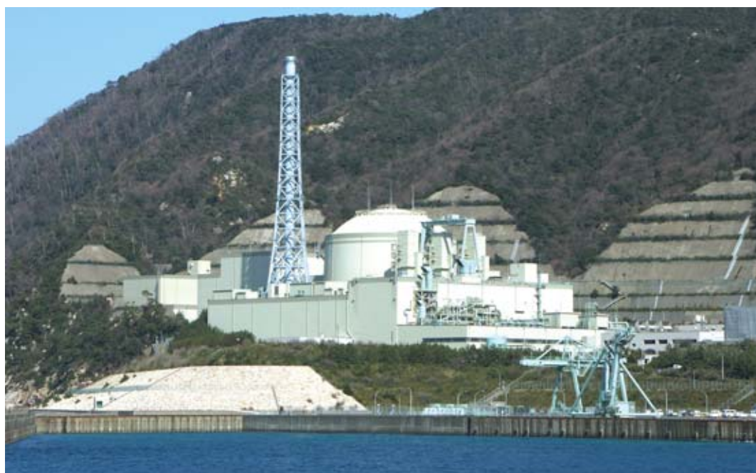
The Monju experimental sodium-cooled fast reactor, in Japan. Currently closed down for alterations, it is due to be recommissioned in 2009. It is planned to irradiate, in this reactor, a minor-actinide charge-bearing fuel assembly in 2020, under the aegis of the GACID program.
