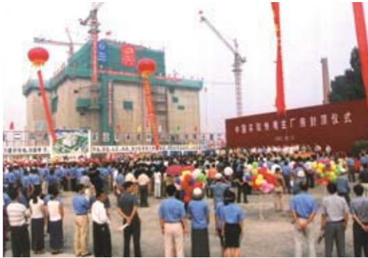
The Chinese CEFR (China Experimental Fast Reactor) sodium-cooled fast reactor, undergoing construction. This experimental reactor will be of the integral type, featuring two secondary sodium loops, and will use a mixed uranium-plutonium oxide as fuel. It will have an output power of 25 MWe. Initial criticality is scheduled for 2009.
