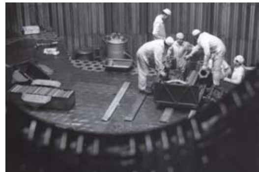
Assembling the graphite stacks in the EDF3 reactor, at Chinon (France), in the mid-1960s.
