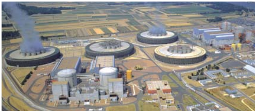
The four PWR units of EDF's Avoine power station, near Chinon (central France), belong to the second generation of nuclear reactors.
