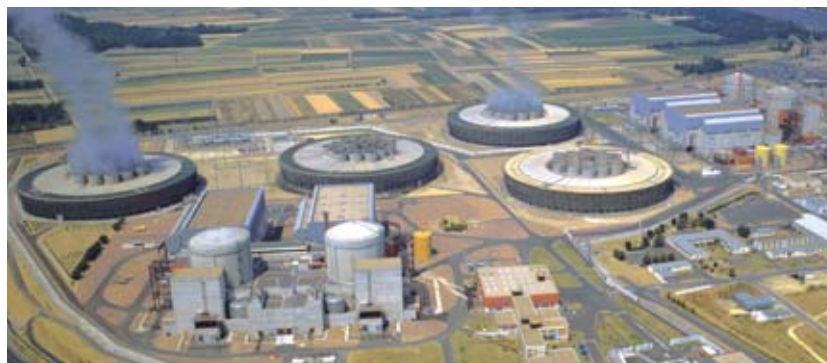
The four PWR units of EDF's Avoine power station, near Chinon (central France), belong to the second generation of nuclear reactors.
