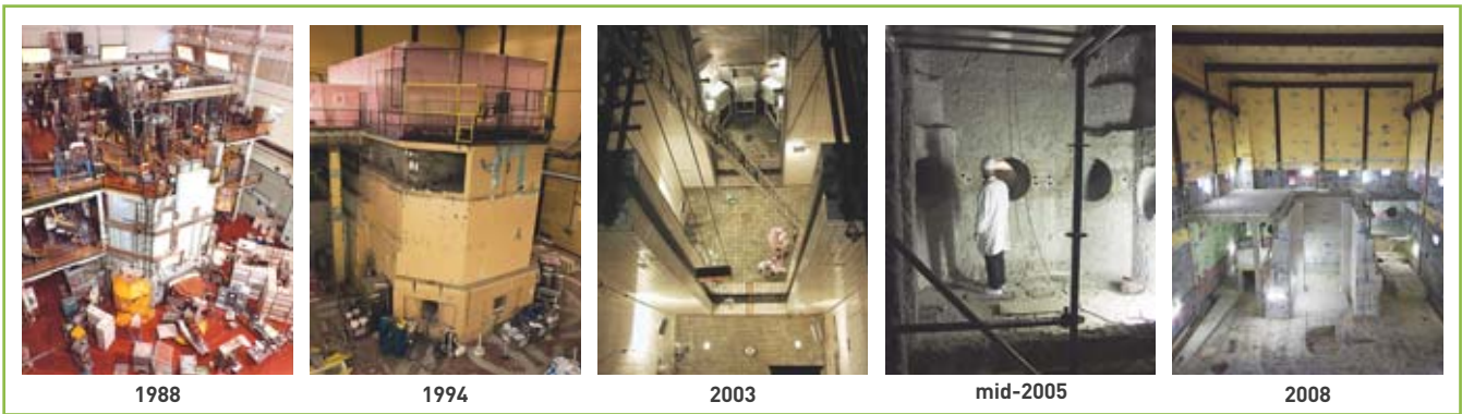
The stages in dismantling of the Mélusine reactor in the CEA Grenoble Center. 1988: the reactor hall in operation; 1994: disassembly of experiments and associated protocols; 2003: reactor pool at the end of cleanup after drainage; mid-2005: final checks on the pool after peeling of the concrete; 2008: reactor hall after removal of the pool block and internal structures (physical state of the BNI at the moment of its delicensing in late 2011).
