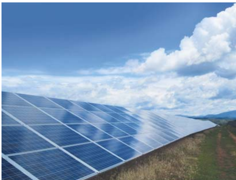
Les Mées photovoltaic solar array in the Alpes-de-Haute-Provence département. Equipped with 105,000 photovoltaic panels over 50 ha, its power output is 24 MWp. Production is 34 GWh, or the equivalent of the annual consumption of 22,342 inhabitants. This array entered service in February 2011.
