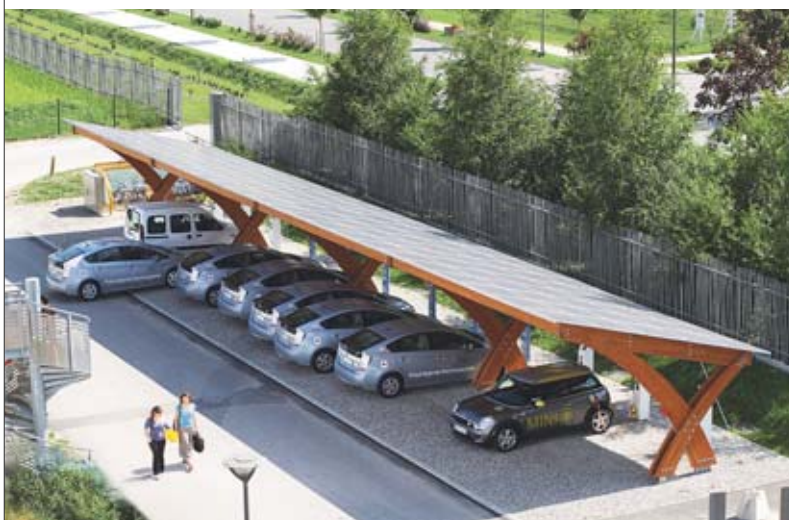
Solar car park on the Ines site in Chambéry (Savoie département ). The wooden sun shelter is covered with photovoltaic panels. It offers 12 parking spaces, i.e. a surface area of 150 m 2 . The station is equipped with 12 recharging terminals.
