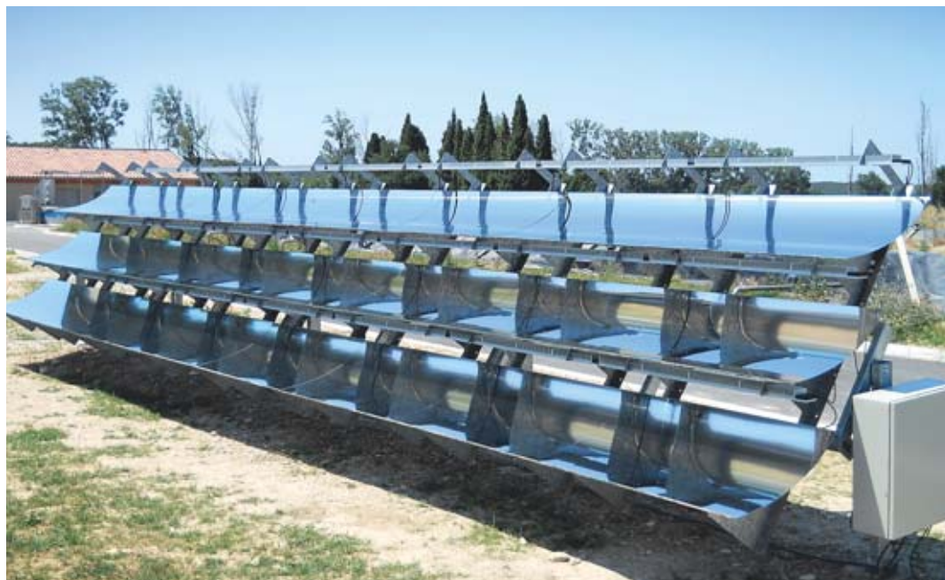
System of Medium Concentration PhotoVoltaic panels (MCPV) from the Axiosun company deployed in the south of France. MCPV systems use single-axis trackers, here oriented East-West. The mirrors, which concentrate the light on the CPV modules, are clearly visible. They are attached to finned heat dissipation devices to limit the temperature rise on the cells.
