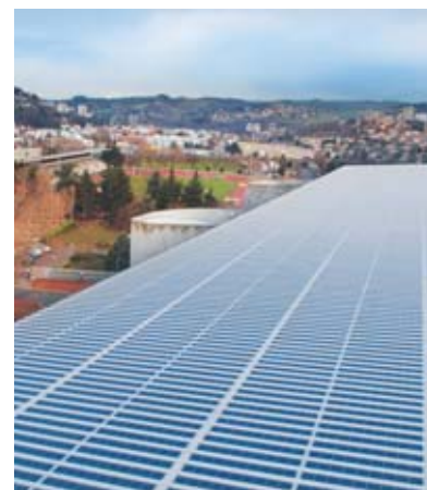
Les Mées photovoltaic solar array in the Alpes-de-Haute-Provence département. Equipped with 105,000 photovoltaic panels over 50 ha, its power output is 24 MWp. Production is 34 GWh, or the equivalent of the annual consumption of 22,342 inhabitants. This array entered service in February 2011.
